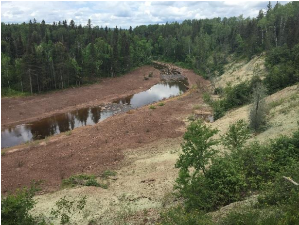
The Knife River GLC/CWF project site, constructed in summer, 2015.
