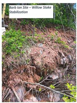
Barb Ion – Flood restoration questionable. Trees and plants not thriving. Owner not providing buffer to bank failure area. Sent letter outlining sources of damage, asking for buffer and recommended installation of rain barrel. Gabions placed by owner appear to be functioning well. Possible Opportunity for Cost Share
